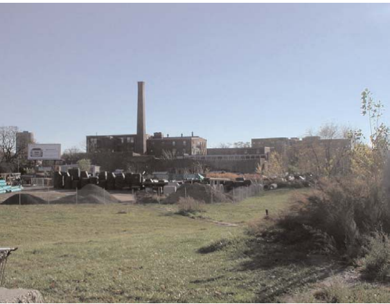
Site Before Redevelopment Source: Boston Redevelopment Authority
