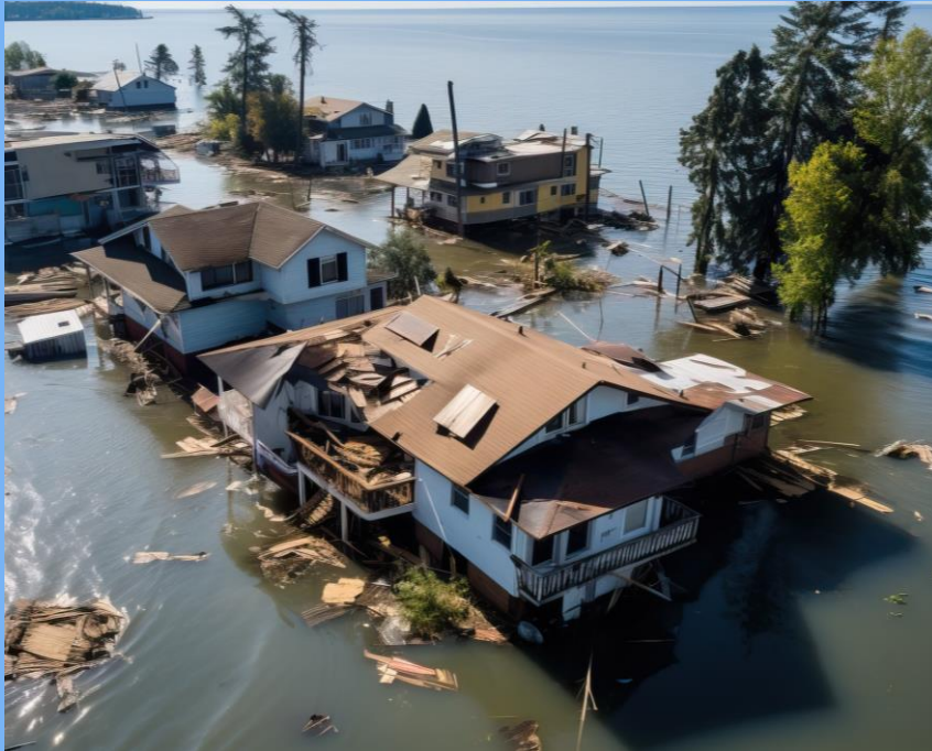
Structures damaged by flooding
