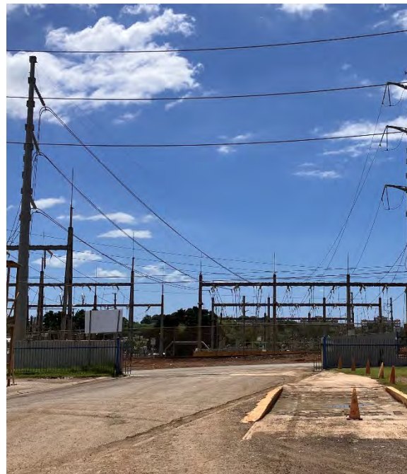
Mayaguez Landfill. Photo by Angela Ortega Pastor, NREL 89451
