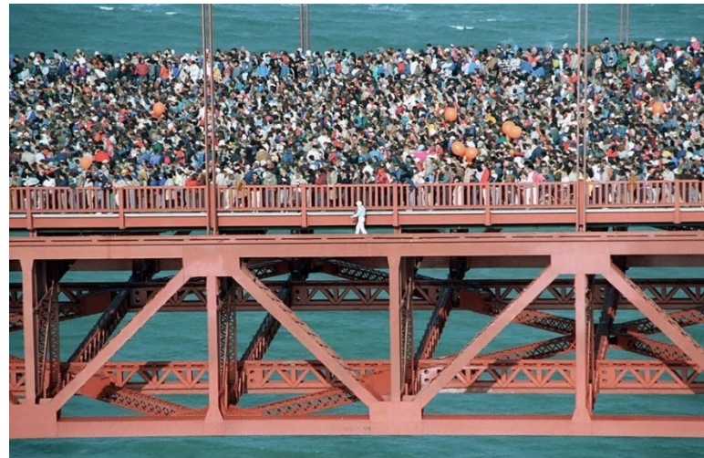
Golden Gate Bridge on its 50th Anniversary in May 1987: a classic example of live loads overload AP Photo / Doug Atkins
