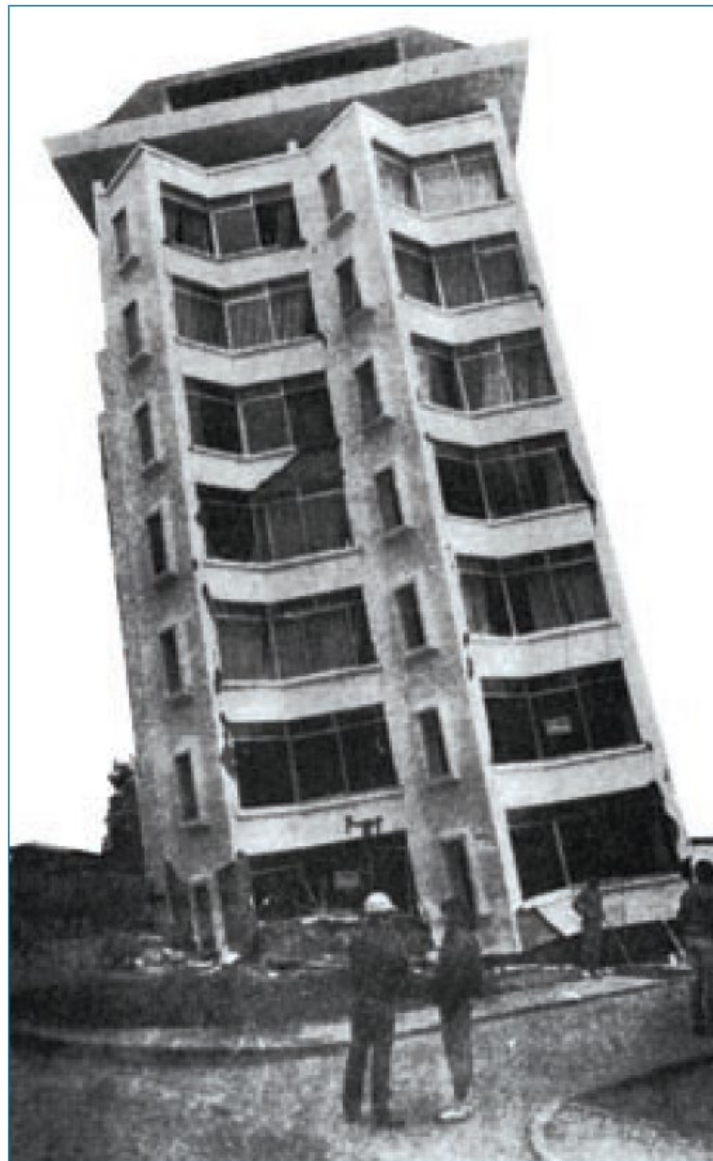
Chile Earthquake 1985 (building in Viña del Mar)
