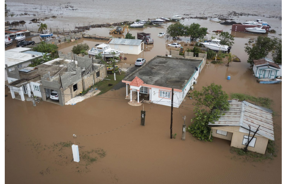
Flooding from Hurricane Fiona in Puerto Rico Source: AP News
